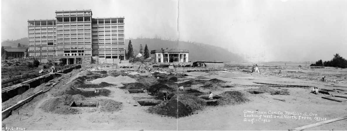
Figure 2. Montgomery Ward building under construction, c. 1920, looking west. Note the remains of the former Oregon State Building to the right prior to its demolition. The work in the foreground is for the American Can Company building [now occupied by ESCO]. (Oregon Historical Society Neg OrHi 105077)
